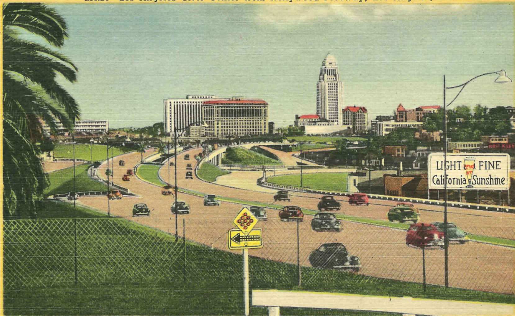
LA.23—Los Angeles Civic Center from Hollywood Freeway, Los Angeles, California
